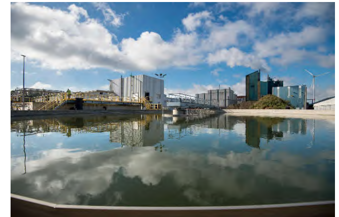
Umicore water treatment installation in Olen, Belgium
